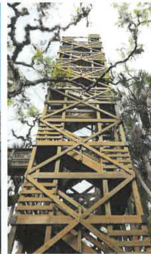
OAK OPENINGS OBSERVATION TOWER
